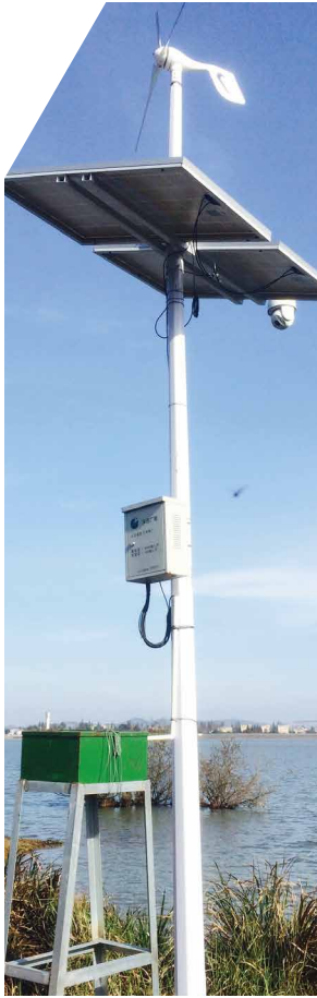
Water Conservancy Zhejiang China
